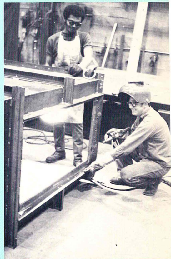
Right — Lloyd Vaughn and Gene Rumfeld finish welding the housing.
